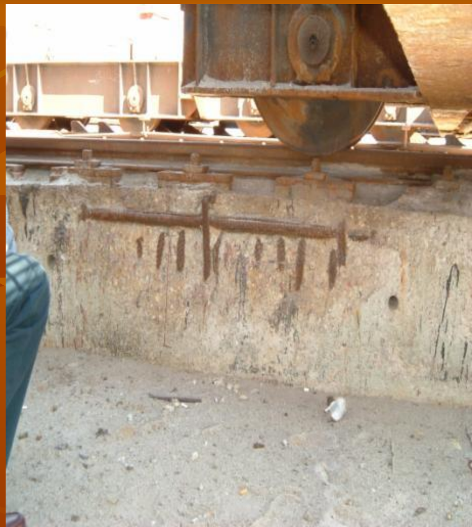
Shahid Rajaei Port Damage to Rail Foundation
