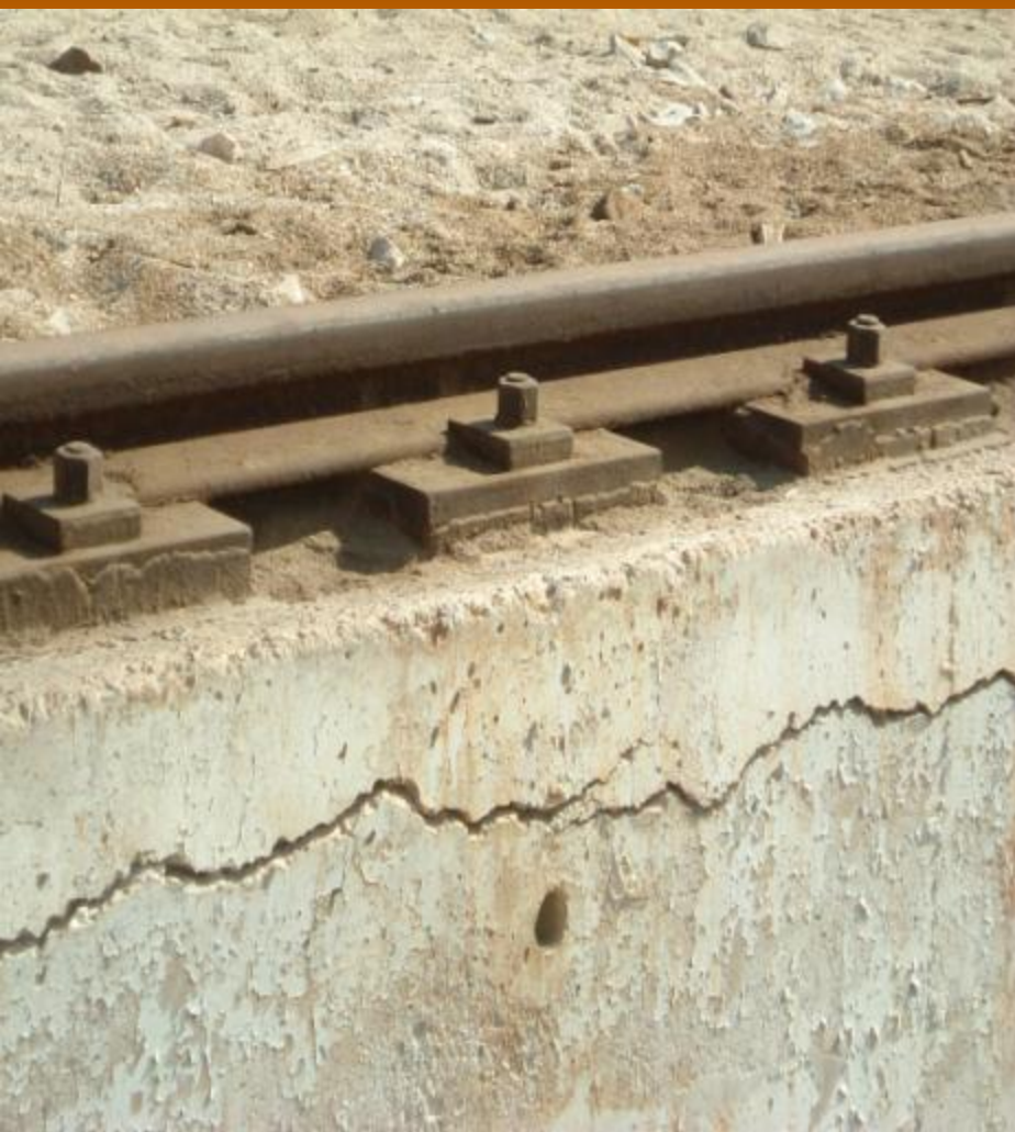
Shahid Rajaei Port Damage to Rail Foundation
